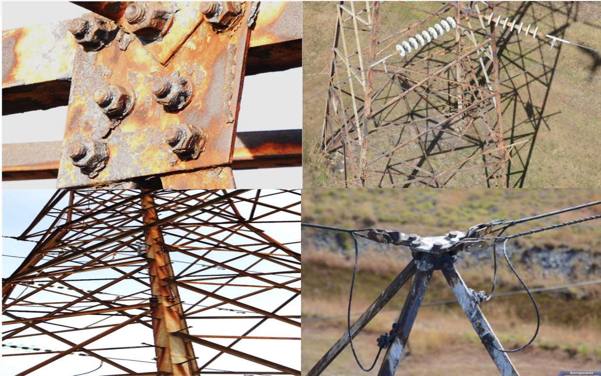
Figure 3: Typical tower condition
