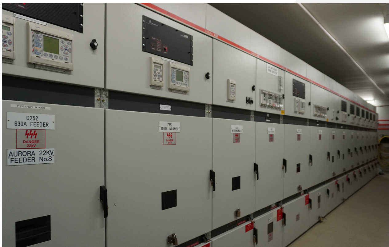
Pictured: Medium voltage distribution equipment
