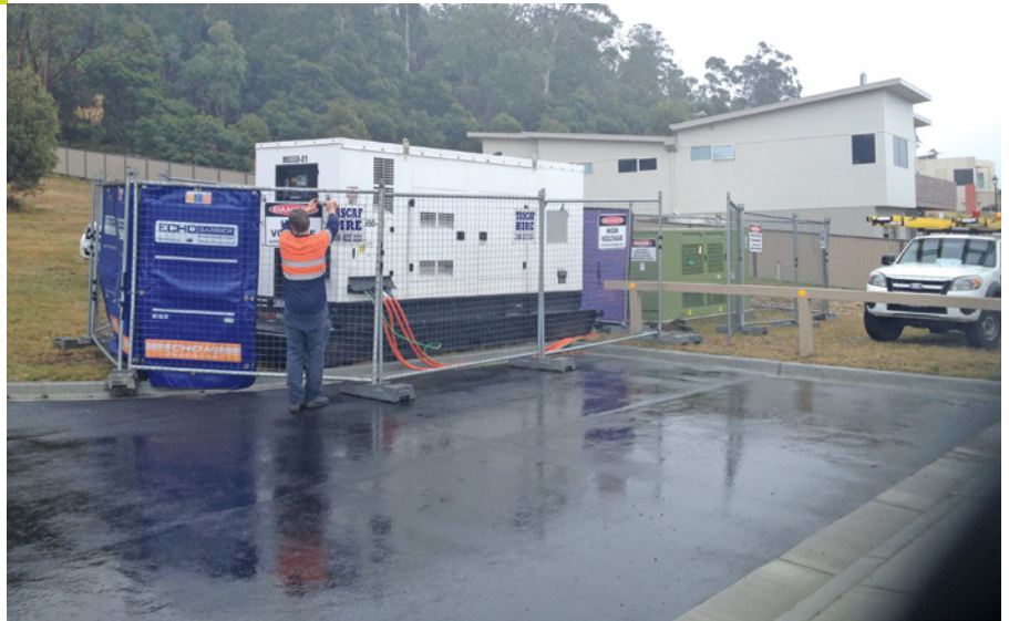
In residential areas baffles can be used to reduce noise generated by equipment
