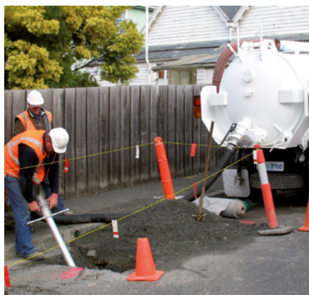
Where possible a licensed liquid waste tanker should be used to pump out accumulated stormwater. Source: Derwent Estuary Program
