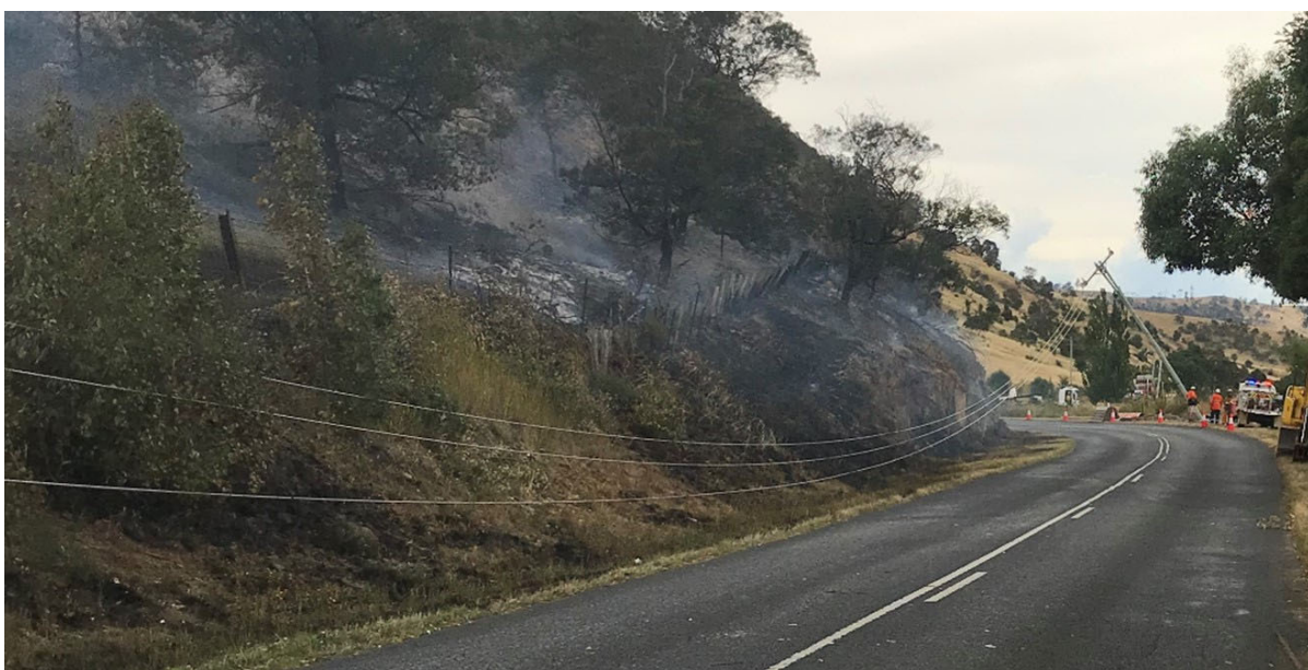
Photo 3: HV conductors touching vegetation between poles 199359–199360
