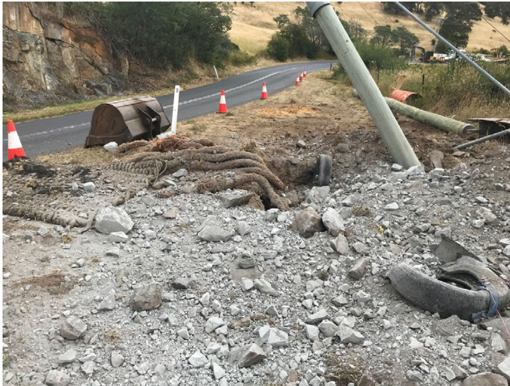
Photo 5: Scene immediately after blasting
