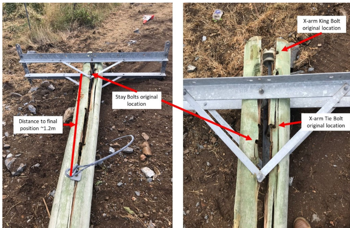
Photo 8: Pole 199360 – post blast after recovery
