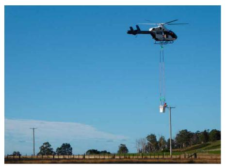
Trialling our new Helicopter Elevated Line Maintenance (**HELM**) system. Photo courtesy of TasNetworks Team-member Mark Wright
